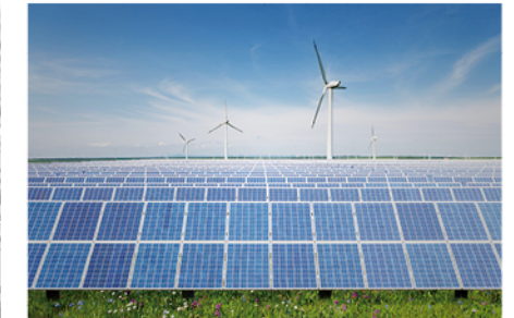
光伏设备 Photovoltaic equipment
